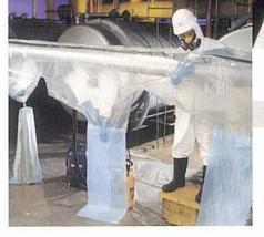
**QuickTwist 1-2-3** is available in Grayling's patented **extended-run** design that set the industry standard for efficiency in removing long runs of pipe insulation.
