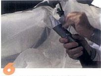
Fill the sprayer with the surfactant. Follow the manufacturers instructions for details on mixing and using the surfactant. Insert the HEPA vacuum and wetting wand of the pump sprayer through the entry ports. Seal each to the entry port socks with duct tape.
