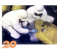
Remove all stubs remaining, starting a the collar, slitting the top of the stubs free while folding inward into an asbestos disposal bag.
