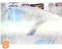
Seal any leaks with additional duct tape and loosen the collar. Repeat this procedure for each glovebag chamber before working in it. Should the glovebag become punctured during any part of asbestos removal, quickly repair it with duct tape.
