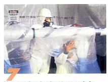
Now test the glovebag tape seals for integrity using the smoke test kit. First, tightly cinch off the collar in the first compartment using the strap or duct tape. Insert the smoke generator through one of the entry ports and introduce just enough smoke to fill the chamber. Remove the smoke generator and seal the entry port with duct tape. Gently squeeze the bag and watch for escaping smoke at the tape seals.
