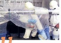
Lift the insulation off the pipe and lower it to the bottom of the bag. Be sure to remove the insulation that extends into the collar. Typically, insulation attaches to pipes in semicircular segments. Insulation is typically installed in 3-foot or 1-meter sections. So, if you are careful to find the seam, you can easily remove the insulation intact. Unless the insulation is severely deteriorated or friable, these segments usually come off easily.
