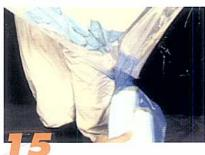
When empty, simply twist off the contaminated chamber just below the pipe, between the work area and the debris chamber, and tightly wrap the twisted section with duct tape.
