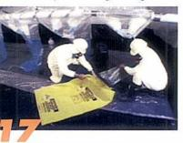
nmediately place the contaminated hamber into a properly marked sbestos disposal bag. You're now eady to move to the next chamber and epeat the process. The Quick-Twist ebris chamber is a major approvement over earlier glovebag esigns. Early designs were too wide at the debris chamber, which made this ritical process cumbersome.
