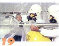
Then remove the last chamber of the glovebag using the previously described procedures.
