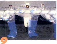
ou are now ready to remove the insulation Put your hands and arms into the first glove/sleeve assembly. Senerously wet the insulation with surfactant. Using tin snips cut any anding or wires that hold the jacketing in place. Carefully remove the jacketing, specially if it is made of metal. The harp edges can cut the glovebag. Fold the jacketing inward so no sharp edges are exposed. Some contractors insert woven bags to hold the jacketing inaterial and protect the glovebag.
