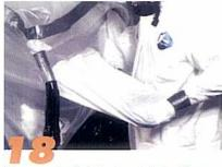
Once you've finished work in the final chamber of the QuickTwist extendedrun glovebag, you have to remove the tools. Grasp them with one of the glove/sleeve assemblies, and pull the sleeve inside out.
