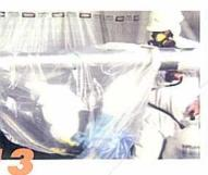
the pump sprayer with encapsulant is spray a generous coating of it onto pipe and inside the glovebag. This is down any residual asbestos fibers. We pass the tools into the next work umber
