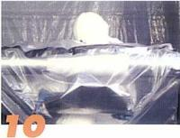
Gently lower the jacketing to the bottom of the bag. Wet down the insulation again with surfactant. If the insulation is firmly attached to the pipe, it may be necessary to use a flexi-wire saw to cut through the insulation. The unique shape of the Quick-Twist glovebag allows you to easily remove whole sections of pipe insulation intact and safely detach the debris from the pipe.
