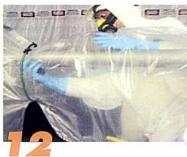
One of the benefits of extended run Q glovebags is the ability to work a continuous piece of pipe ... reaching between chambers. Thoroughly scrap or chip off the remaining asbestos usin a scraper. Once the insulation has been removed, scrub the pipe clean using the brush and surfactant.
