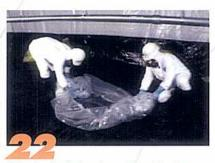
After the last chamber of the glovebag has been taken down and safely disposed of, proceed with clean up and decontamination. Fold the drop cloth inward and place it in an asbestos disposal bag. Be careful not to spill any material that may have fallen during the removal process. Seal up all asbestos disposal bags and discard them in accordance with all regulations. If a decontamination unit has been set up, follow all applicable procedures.
