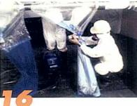
While the vacuum is running, detach the wetting wand and seal the port with duct tape. Deactivate the vacuum and cut the chamber away from the pipe through the center of the taped area. By cutting through the center of the tape you are maintaining an airtight seal, and preventing fiber release. Next, remove the vacuum wand from the glovebag and reseal the port with duct tape.
