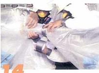
The next step is to seal off the contaminated chamber. Tightly wrap the collar around the uninsulated section of pipe using duct tape or strap. Activate the HEPA vacuum evacuating the air from the glovebag.
